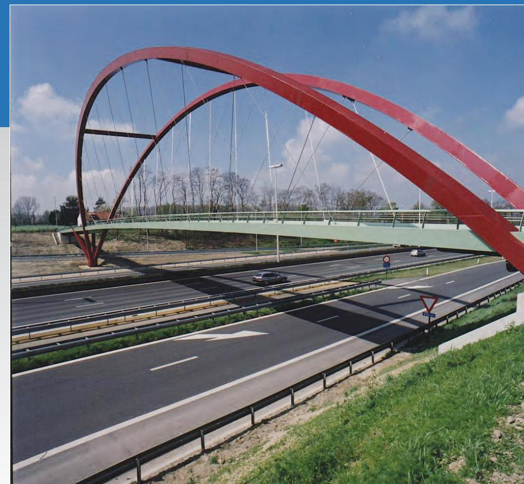
with a fictive E-modulus). Because the linear calculation resulted in compression in the tension bars a non-linear calculation was needed. Because of the light and slender character of the bridge there was also need to calculate the eigenvalues / frequencies of the bridge in order to check if there were risks of vibration under live load or wind actions.
